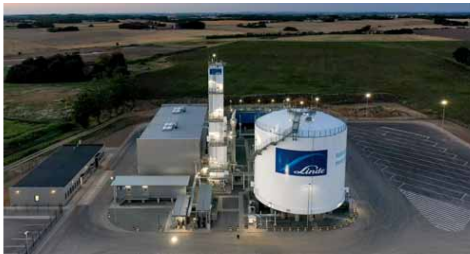
Linde's FLEXASU plant in Denmark, designed to operate and store products when wind energy is abundant and less costly, meets the entire demand for Denmark. Credit: Linde
